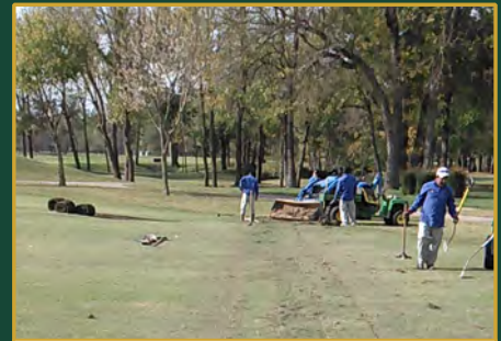
Leveling Of Fairway on #18
