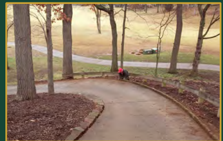
Completed #10 Cart Path/Bed Edging
