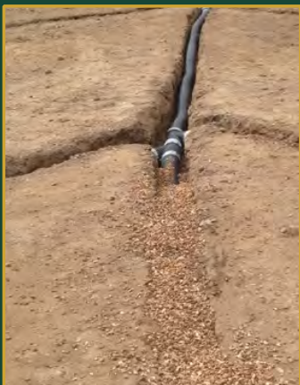
Drainage Repair On #13
