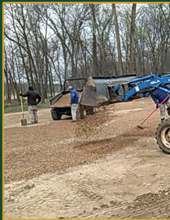
Chipping Green Gravel Layer
